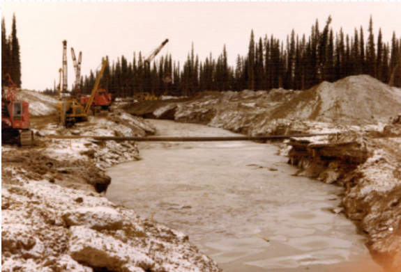
Flow Isolation- Pipe Flume
