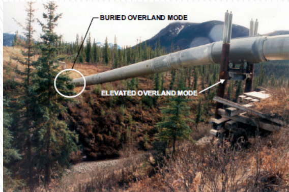
Free span of pipe
