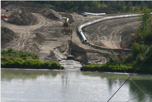
Open Cut – Sauerman Dragline
