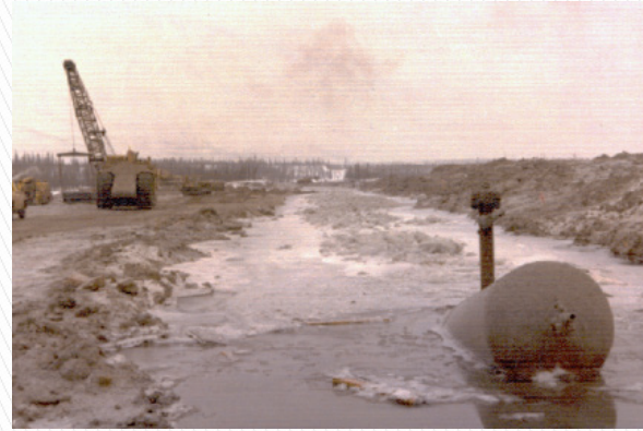
Open cut, wet ditch.
